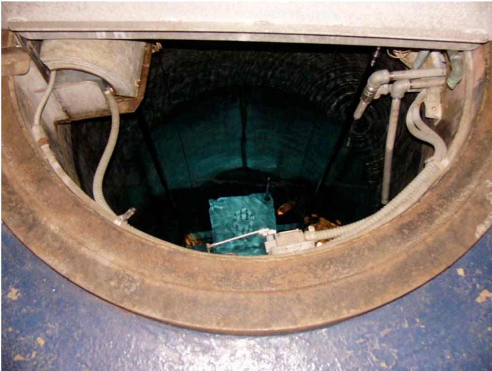
**Figure 3.17** The source at the bottom of the water pool.
